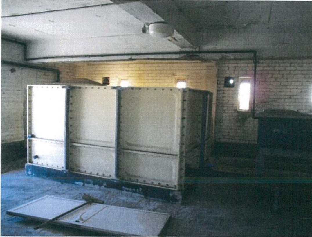
Photograph 9 – View of the tank room.
